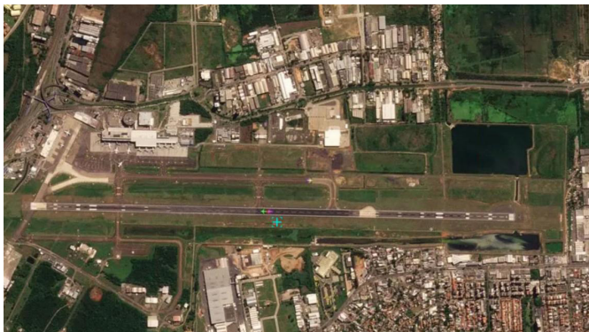
FIG 1: PORTO ALEGRE'S AIRPORT BEFORE THE FLOOD
